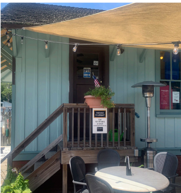
The Ticket Office receives a fresh coat of paint.
